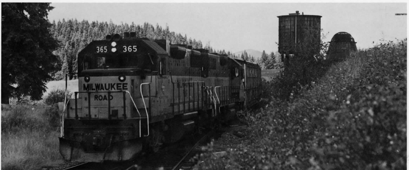
Southbound on the Bovill Run from St. Maries, Milwaukee Road units 365 and 361 are caught passing the water tower at Fernwood, Idaho. Photo taken in 1973 by Ted Holloway.
